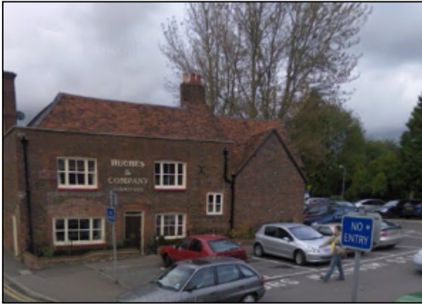
31 Frogmore Street, front (south) elevation
