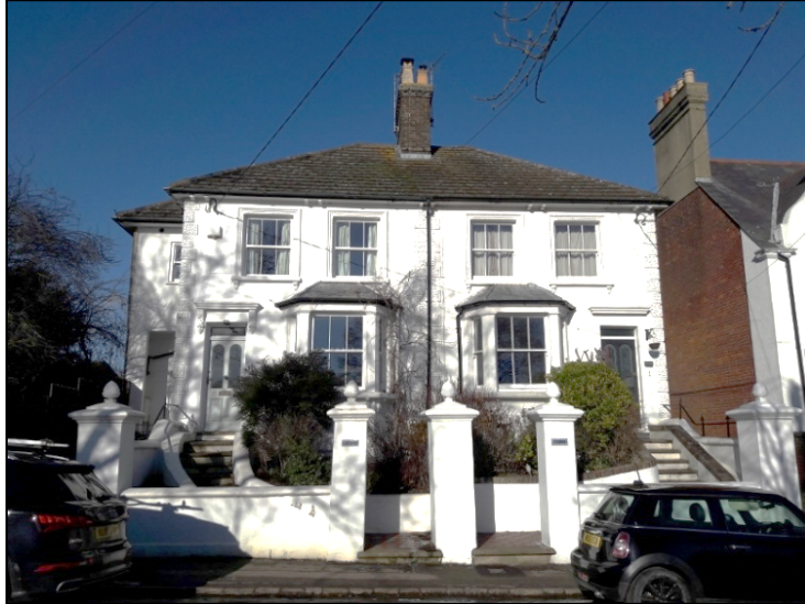
Original boundary walls and piers at Lynwood and Farleigh on Park Road
