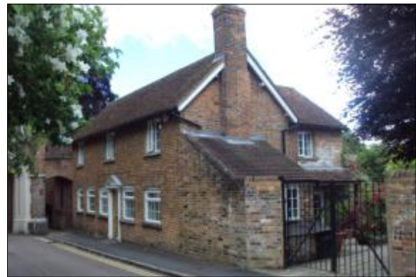
uPVC windows in Vicarage Lodge, Churchyard
